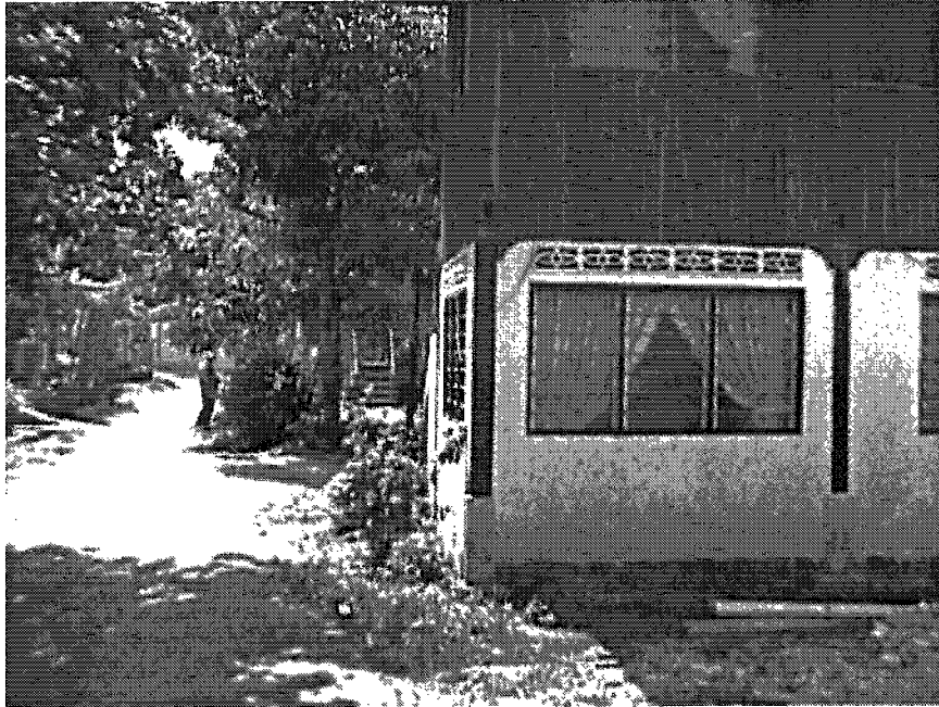
Figure 9 Scenes of Pathways in Kampung Dodol Showing Enclosed Ground-floor Renovations
